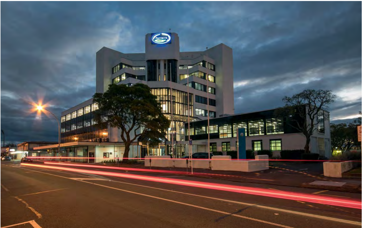
Fonterra House, Hamilton (Wholly owned investment property in New Zealand)
